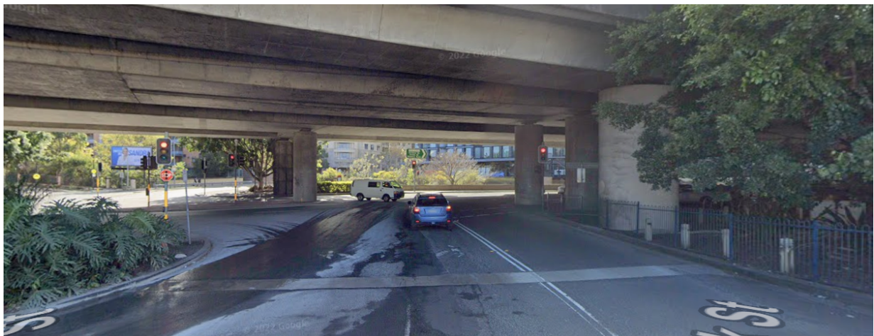
Figure 14: Site Egress via Right Turn into Bank Street
